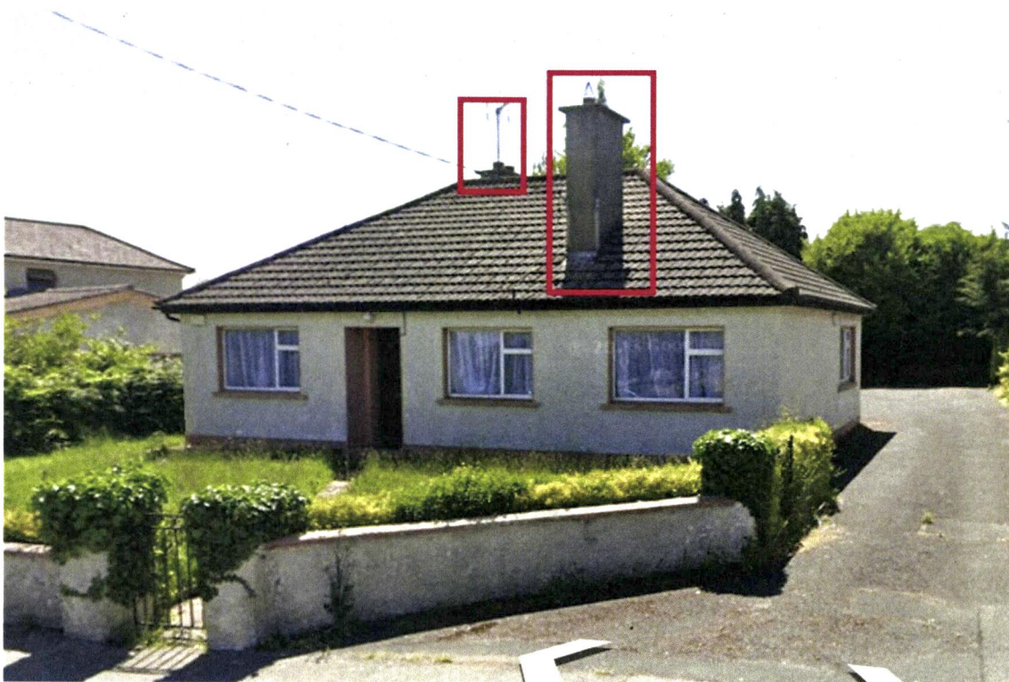
Front View: Removal of chimney
